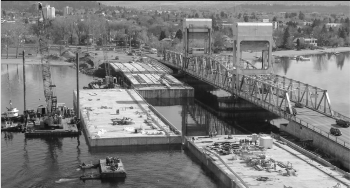
One of the concrete pontoons being moved into position.
