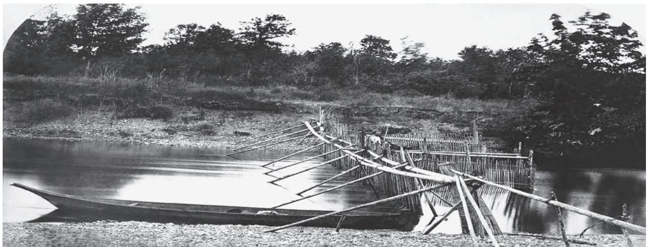
■ This fishing weir on the Cowichan River on Vancouver Island was photographed about 1867. First Nations fishers tailored their weirs for specific locations.
